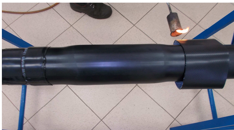
Photo No 44 Shrinking of the heat-shrink band located on the other side of the sleeve
