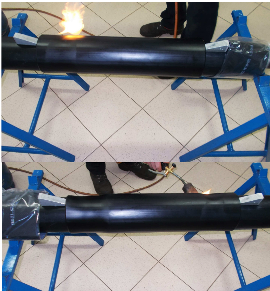
Photos No 29 and 30 Shrinking of the ends of the heat-shrinkable sleeve with LPG blow torch "soft" flame
