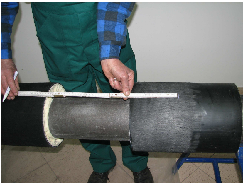
Photo No 25 Marking of the calculated dimensions while determining the location of the edge of the heat-shrinkable sleeve
