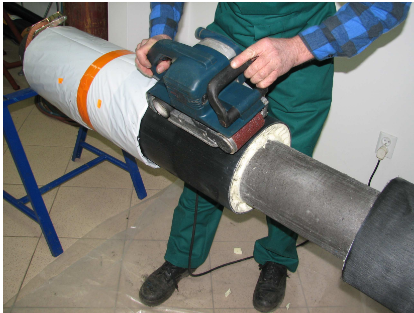
Photo No 23 Sanding of the casing pipe of the pre-insulated element using a belt grinder with sand belt of 50 + 70 grit
