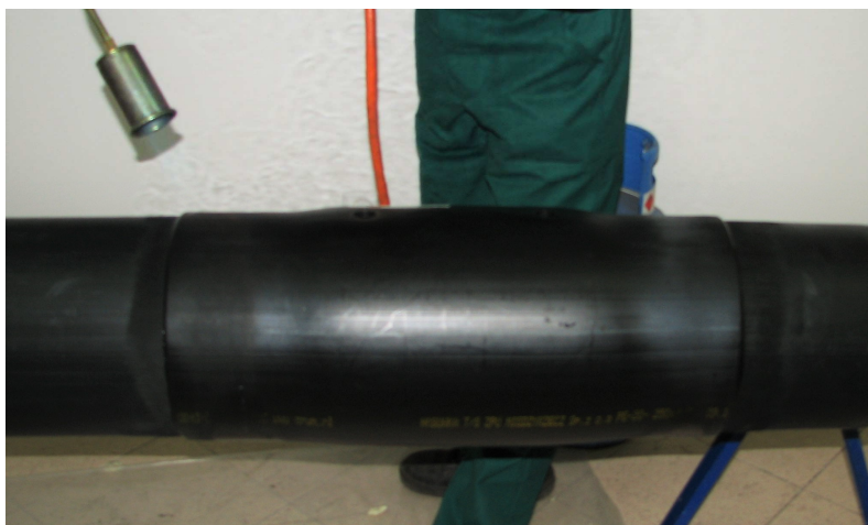
Photo No 37 Heating of the cleaned sleeve and casing pipe to a temperature of ca. 40 °C
