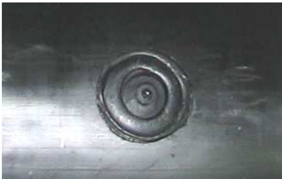
Photo No 60 View of a properly installed welded plug
