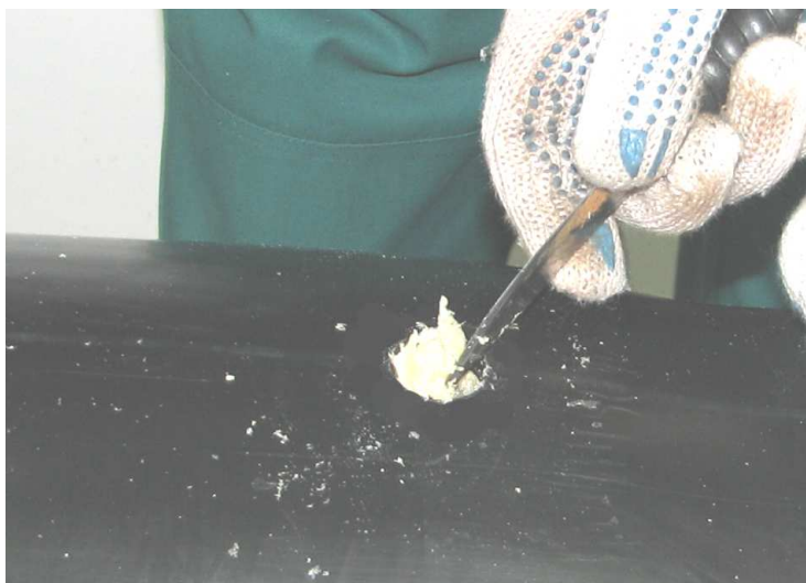
Photo No 54 Removal of PUR foam from the filling holes ca. 5 mm in depth
