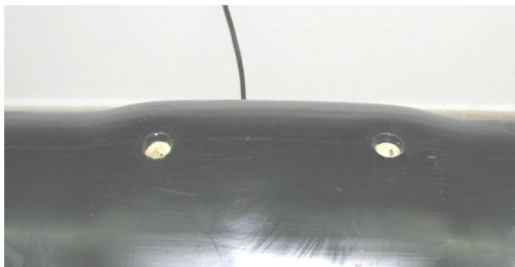
Photo No 56 Cleaning of the filling holes: the place where the welded plugs are installed
