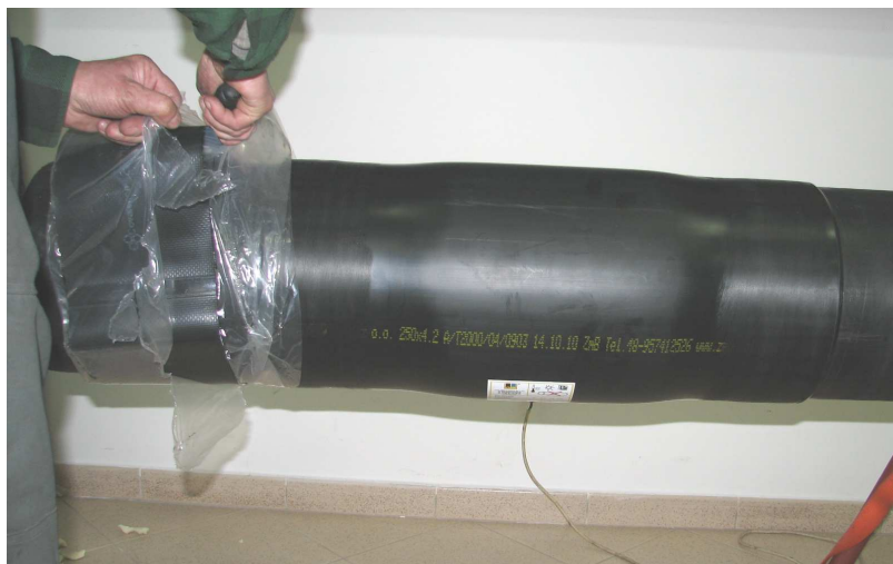
Photo No 38 Putting the heat-shrink bands in place for installation and removing the dirt-protecting foil
