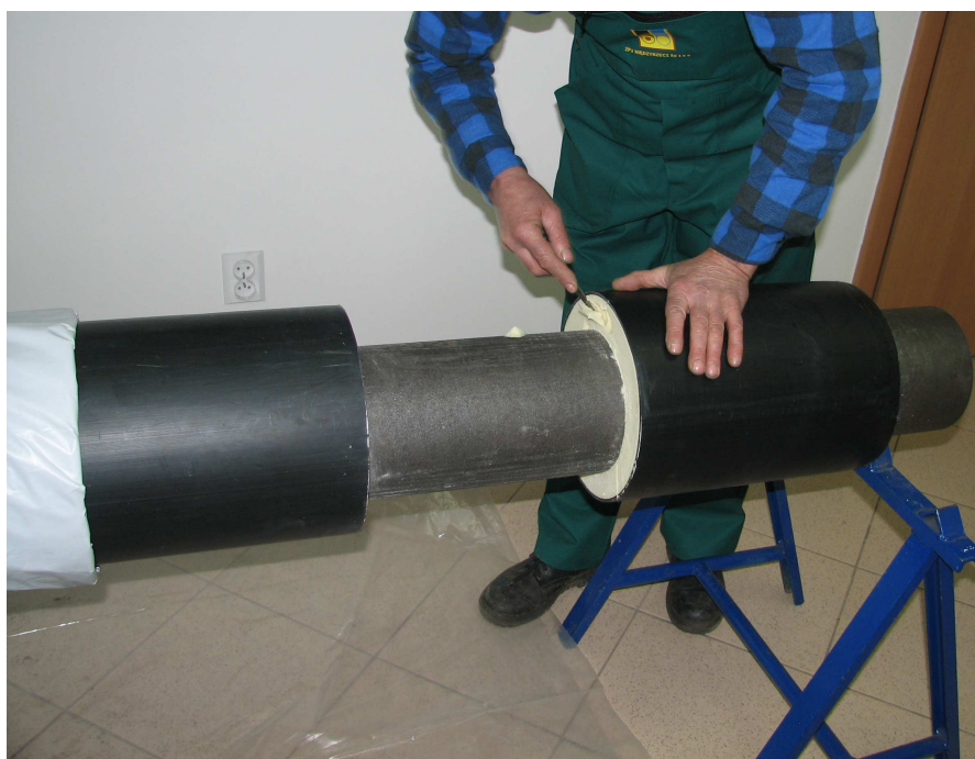
Photo No 22 Removal, using a knife or a scraper, a part of the thermal insulation, the PUR foam insulation, up to 15 mm in depth, from the front of the pre-insulated elements to be bonded
