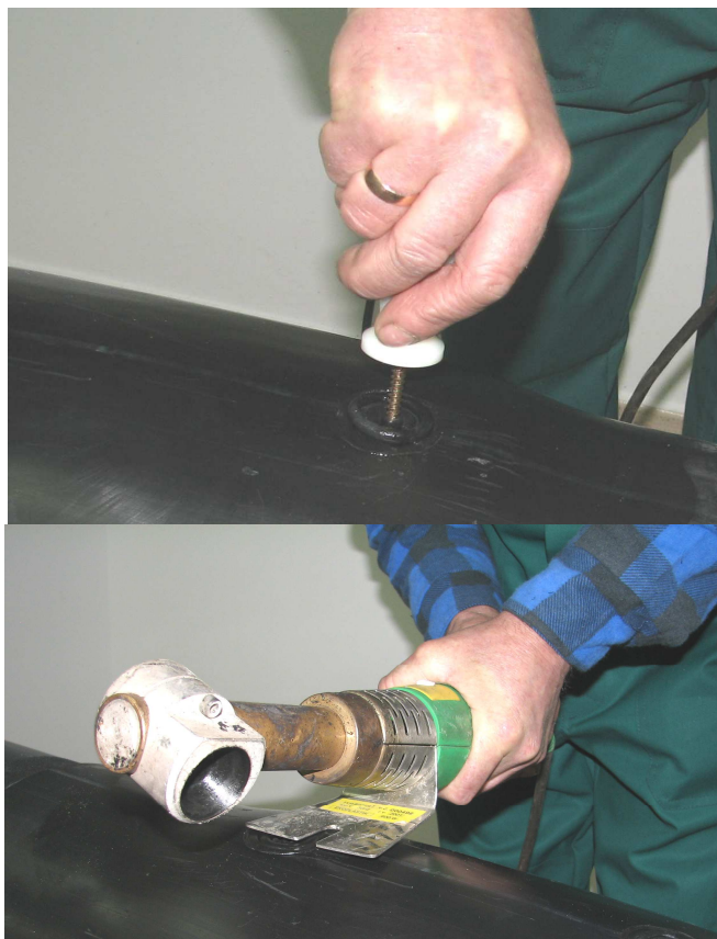
Photos No 58 and 59 Placing the heated plug in the filling hole of the coupling
