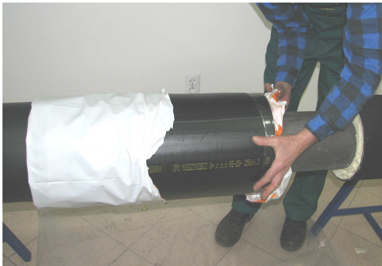
Photo No 26 Removal of the white foil from the heat-shrinkable sleeve
