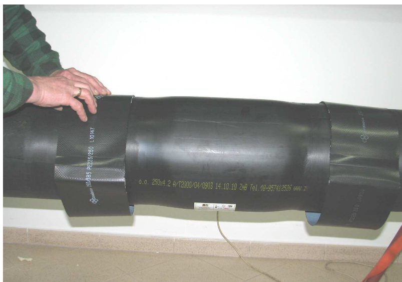
Photo No 39 Placing the heat-shrink bands centrally on the edge of the heat-shrinkable sleeve
