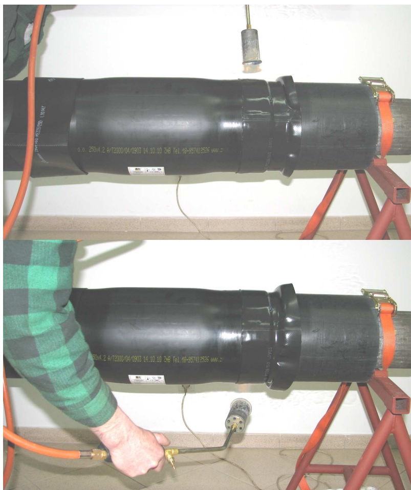
Photos No 41 and 42 Shrinking of the heat-shrink band on the sleeve's side
