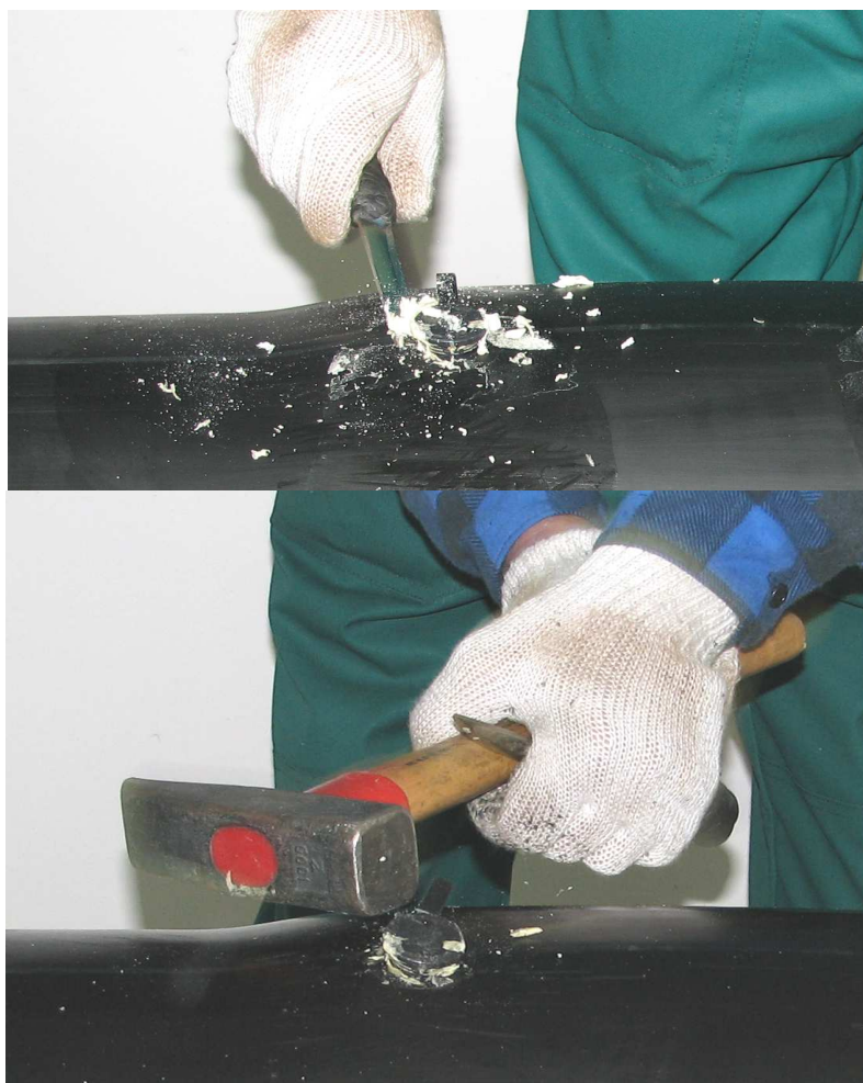
Photos No 52 and 53 Removing vent plugs from the filling holes
