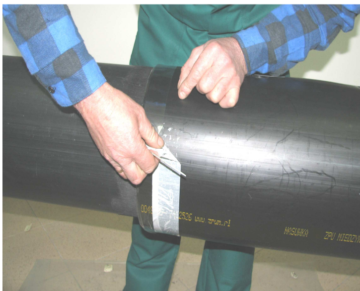
Photo No 27 Removal of the inner foil protecting the adhesive in the heat-shrinkable sleeve
