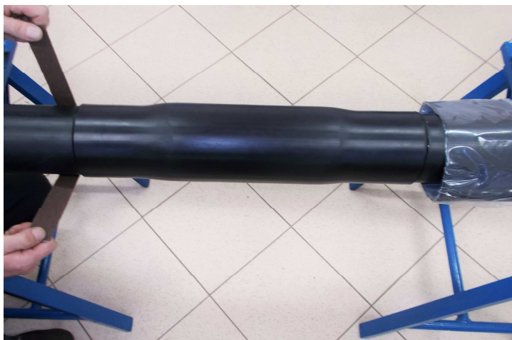
Photo No 36 Hand cleaning by means of sandpaper of 50 + 70 grit of the place of the installation of the heat-shrink bands: the surfaces of the pre-insulated element and heat-shrinkable sleeve casing pipes
