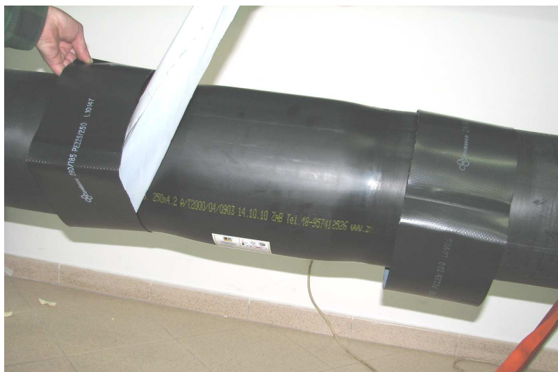
Photo No 40 Remove the dirt-protecting foil from the inner surface of the heat-shrink bands
