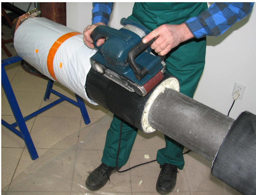
Photo No. 22 Cleaning the casing pipe of preinsulated element using a belt grinder with sandpaper grit 50 + 70
