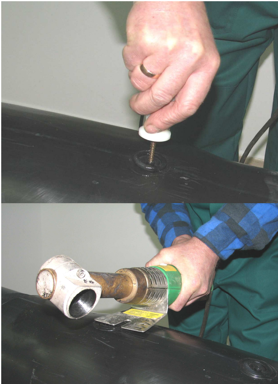
Photos Nos. 46 and 47 The location of the heated plug in the joint's filling hole
