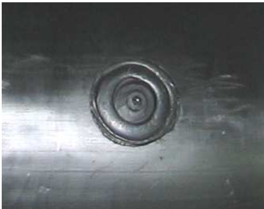
Photo No. 48 View a properly installed welded plug
