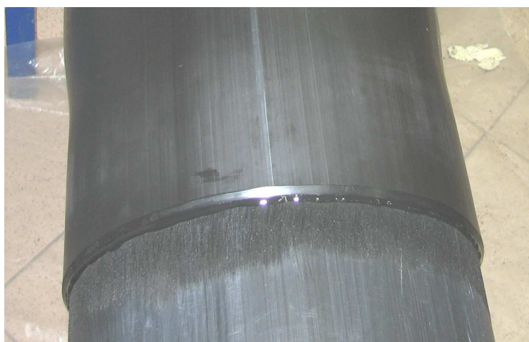
Photo No. 31 View the adhesive bead of glue on the edge of the heat shrinkable sleeve - preinsulated pipe circumference.
