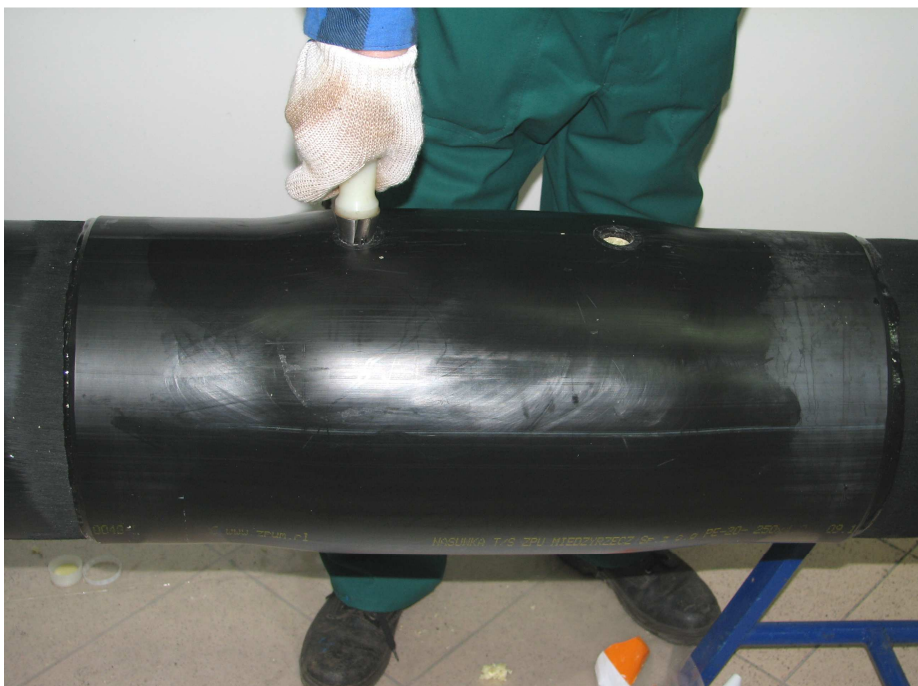
Photo No. 43 Chamfering of filling holes edges using manual conical cutter.
