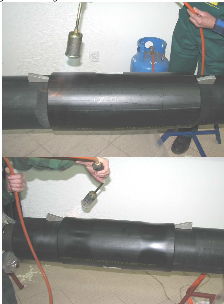
Photos Nos. 28 and 29 Shrinking of heat shrinkable sleeves ends with "soft" flame of burner for liquid propane - butane gas.
