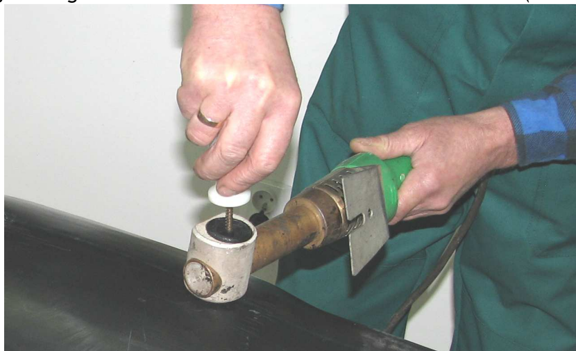
Photo No. 45 Heating to the state of the plastic deformation of the outer edge of the filling hole and the surface of the conical plug with the help of welding machine for plugs
